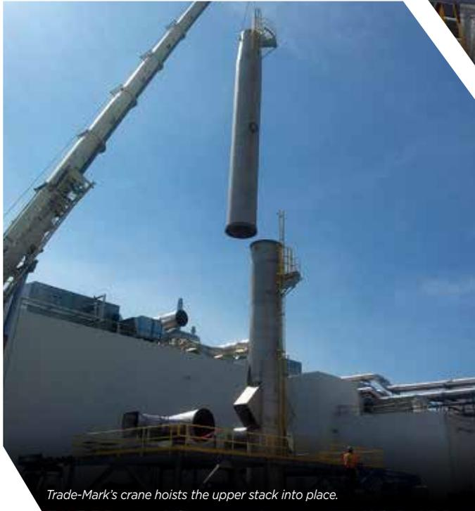
Trade-Mark's crane hoists the upper stack into place.
