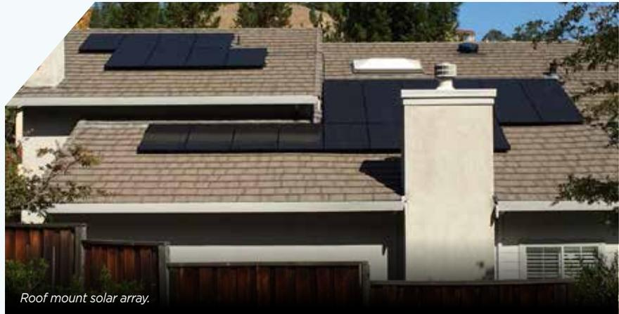
are drawn to the energy savings, environmental benefits and tax breaks. ACS installs roof-mounted panels that tie into the main electrical breaker box.
