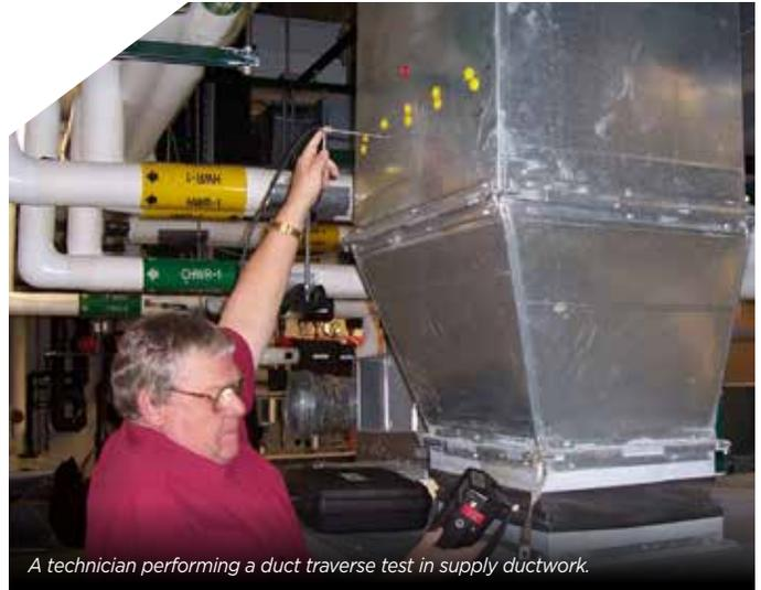
*A technician performing a duct traverse test in supply ductwork.*
