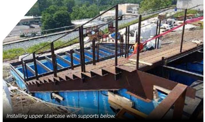
Installing upper staircase with supports below.
