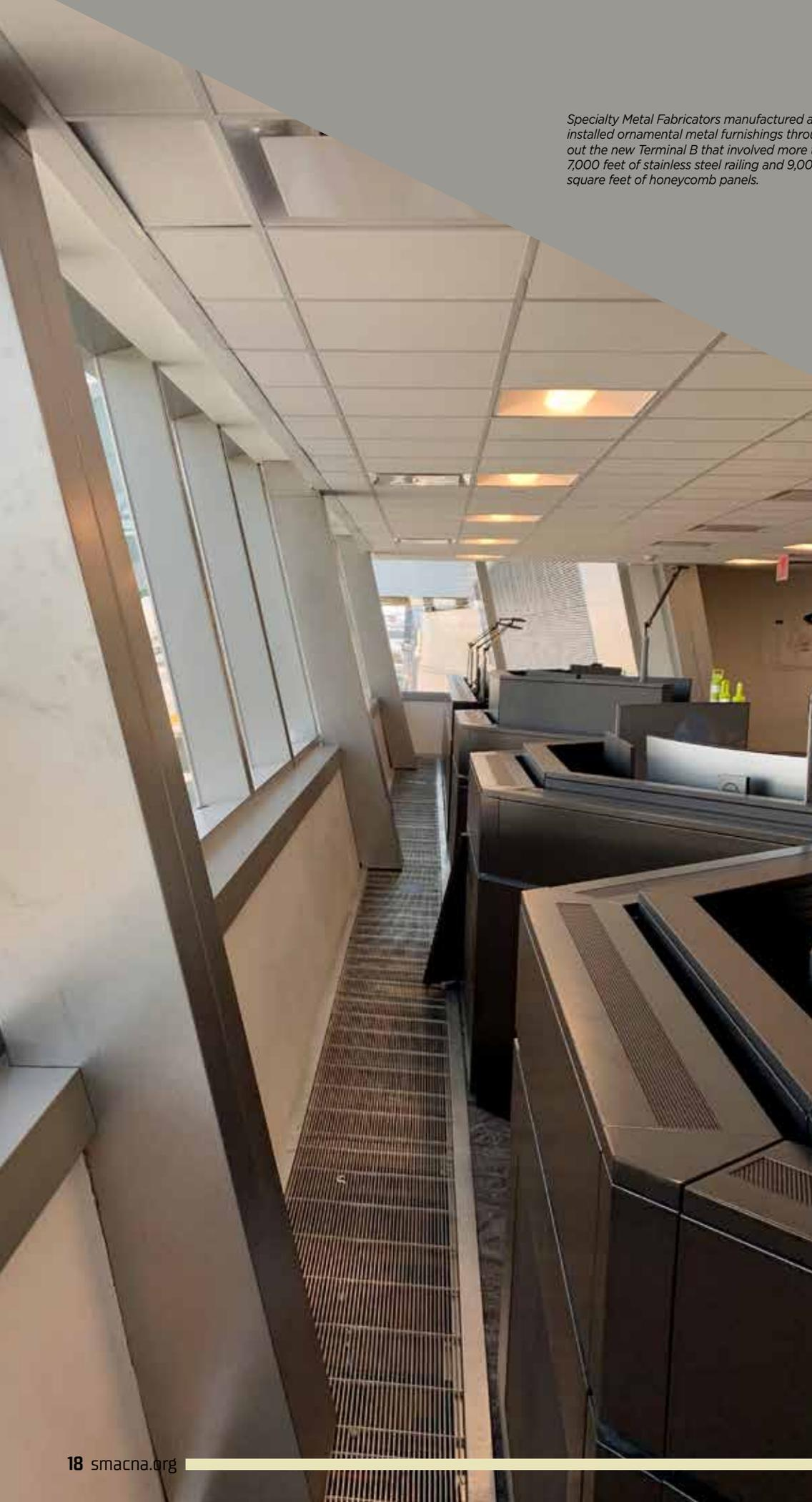
*Specialty Metal Fabricators manufactured and installed ornamental metal furnishings throughout the new Terminal B that involved more than 7,000 feet of stainless steel railing and 9,000 square feet of honeycomb panels.*
