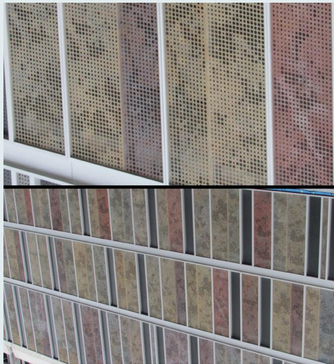
*This picture shows how zinc can be transformed with different oxides.*
