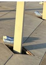
Northern California. All eight structures were 60 feet by 30 feet galvanized finished products, weighing about 4,000 pounds. The structures are mounted on 12-inch by 12-inch tube steel posts anchored into a 10-foot square concrete foundation. Buyers can choose from several pre-painted color schemes to match their properties.
