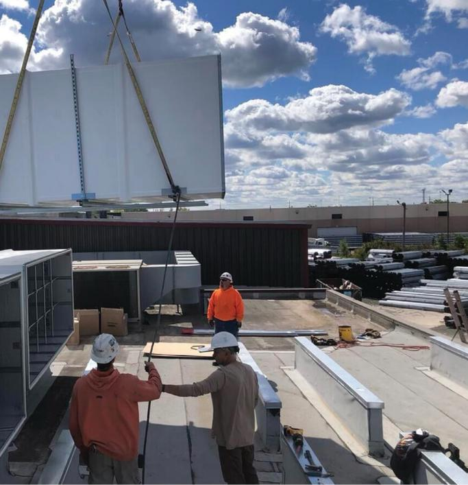
*A large manufacturing company in Harvey, Illinois, needed 170 feet of R-12 ThermaDuct with dimensions of 148 inches by 60 inches. Sheet Metal Werks had to lift and install the pieces onto a rooftop feeding two air units.*
