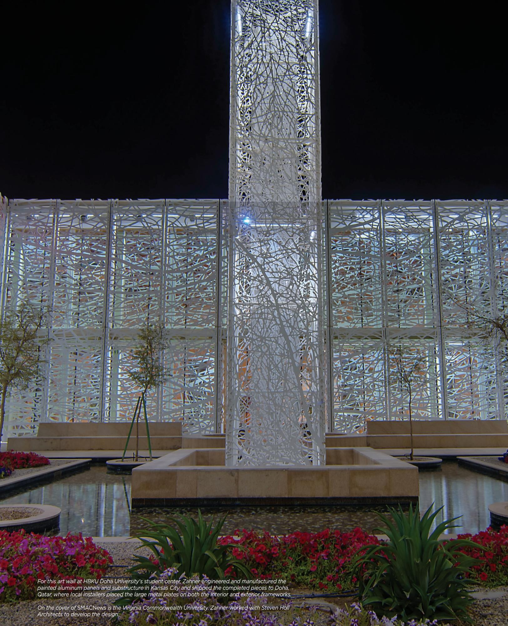
*For this art wall at HBKU Doha University's student center, Zahner engineered and manufactured the painted aluminum panels and substructure in Kansas City and shipped the completed pieces to Doha, Qatar, where local installers placed the large metal plates on both the interior and exterior frameworks.*
